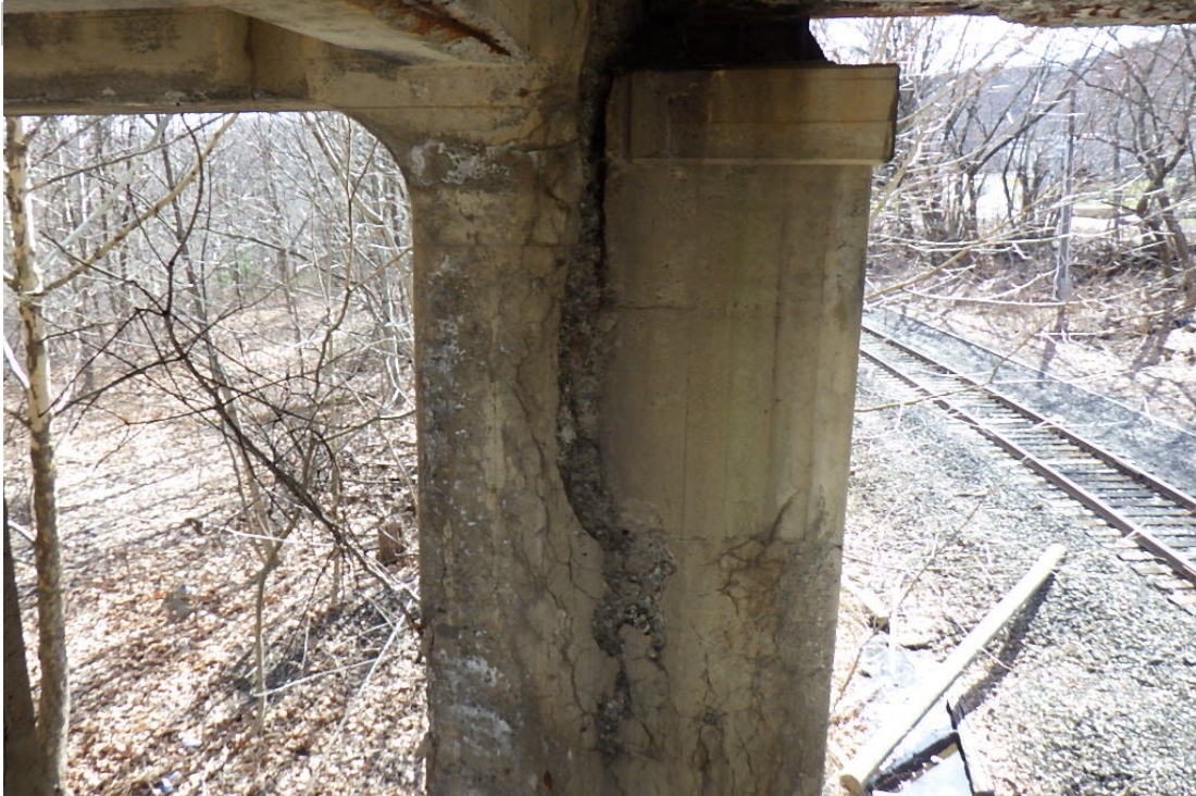
47. Cracks and spall in the left face of Column 2 at Pier 2.
