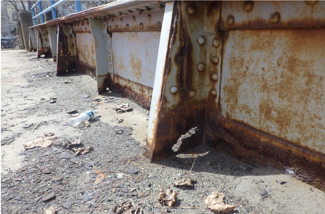
9. Left Girder with 100% section loss to the bottom of the stiffeners and knee brace webs.
