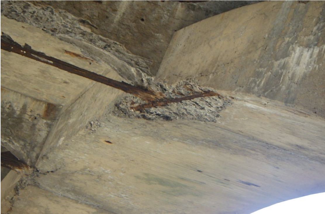
33. Left arch rib at mid-span with spall with exposed rebar.
