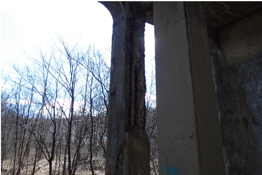
36. Full height spalling with exposed rebar to the right of Column 1.
