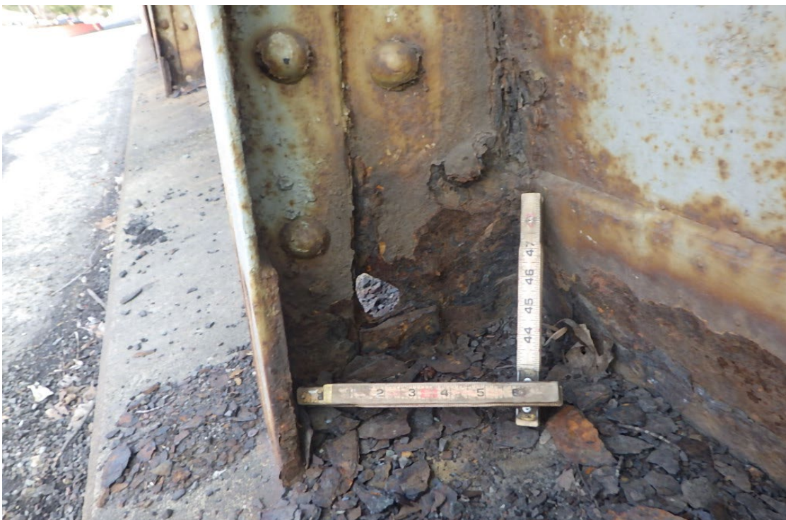
10. Hole in the web of the knee braces for the Right Girder.
