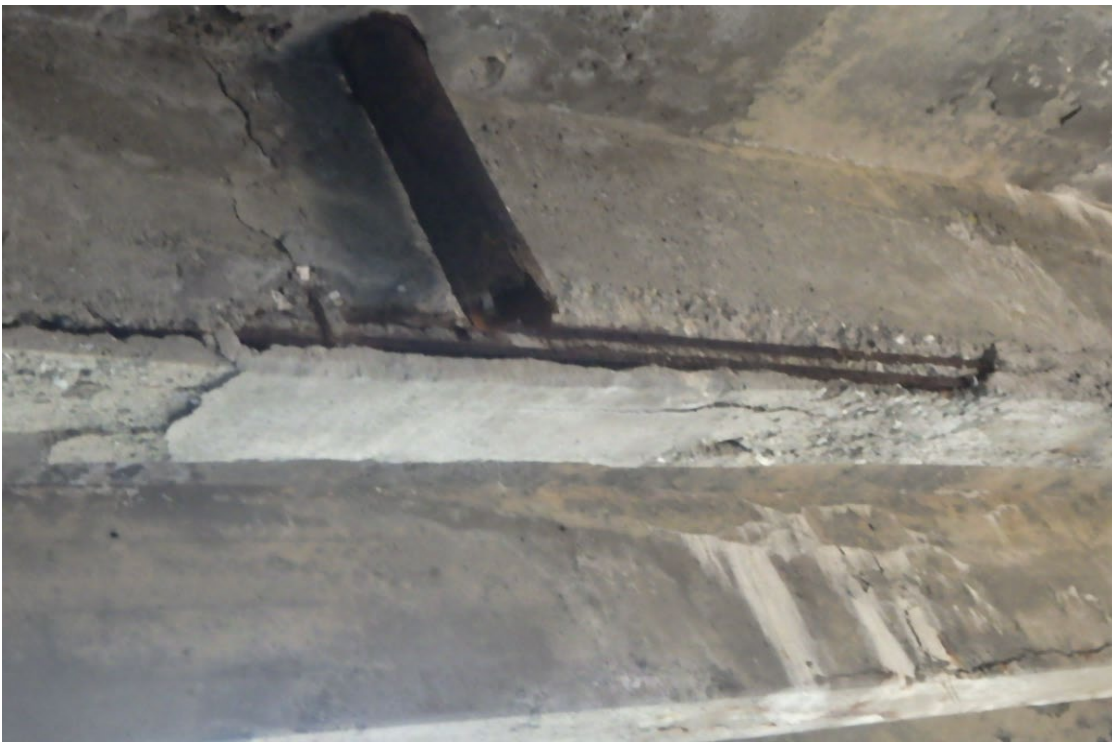
38. Spall with exposed rebar to Beam 2 at the drain outlet in Span 6.
