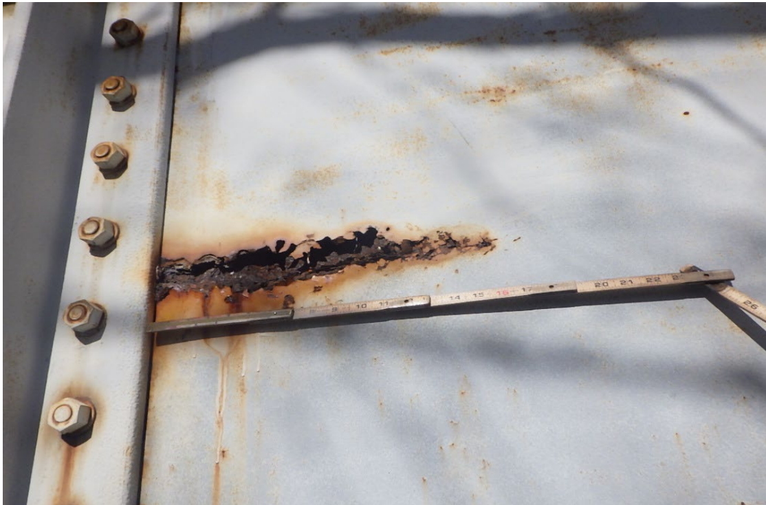
19. Hole in the web of the right girder at the near end.
