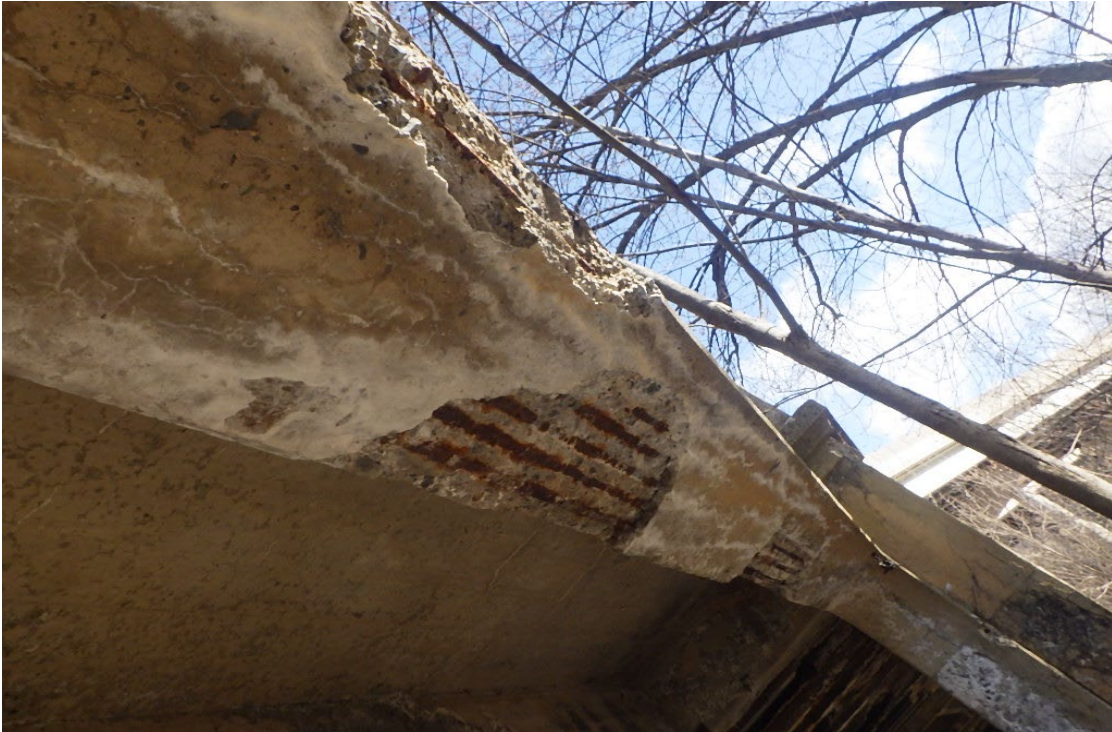
15. Beam 5 in Span 1 with spall with exposed longitudinal reinforcement near mid-span.
