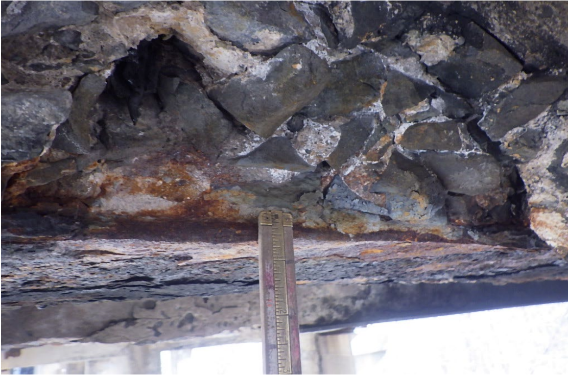
23. Close up of the floorbeam bottom flanges with rust and section loss.
