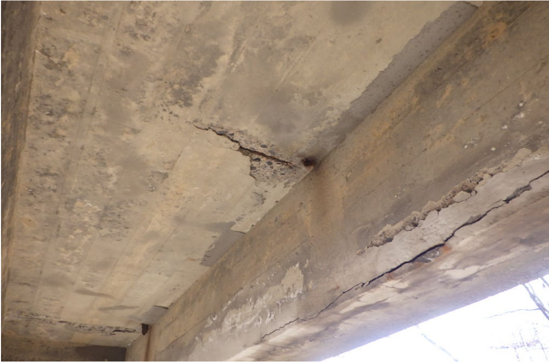
27. Spall with exposed rebar in the underside of the deck, Span 3, Bay 4.
