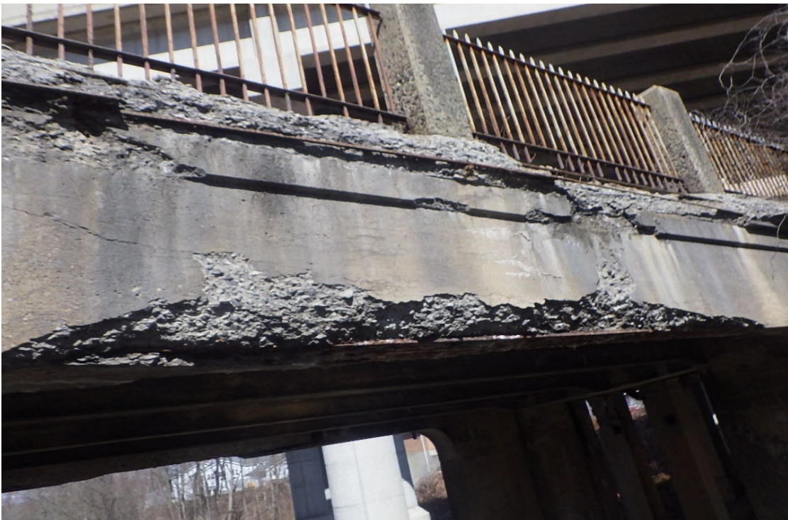
12. Areas of spalling with exposed rebar along the outside edges of the deck.
