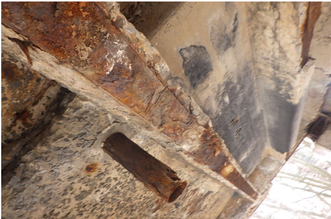
22. Span 2 floorbeams with spalled concrete exposing the bottom flanges.
