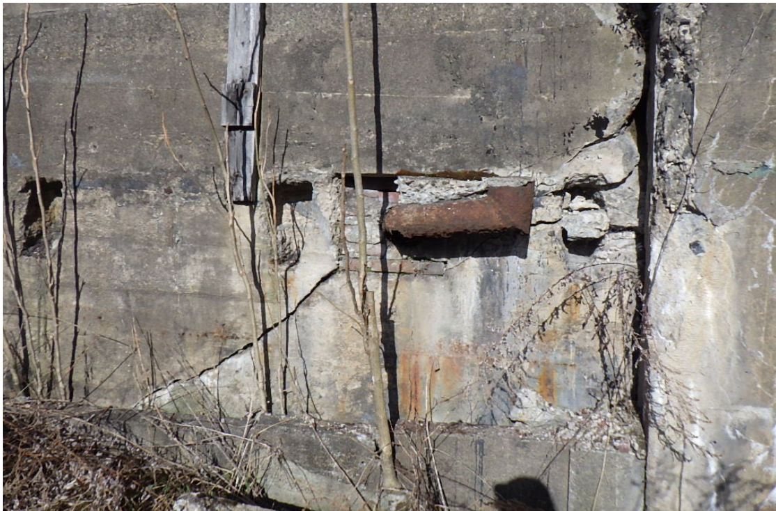
44. Wide diagonal crack in the Near Right Wingwall.
