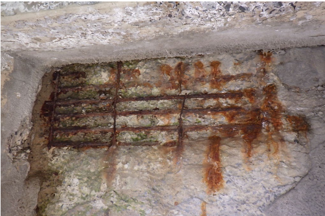
42. Spall with exposed rebar at the left end of the Near Abutment.
