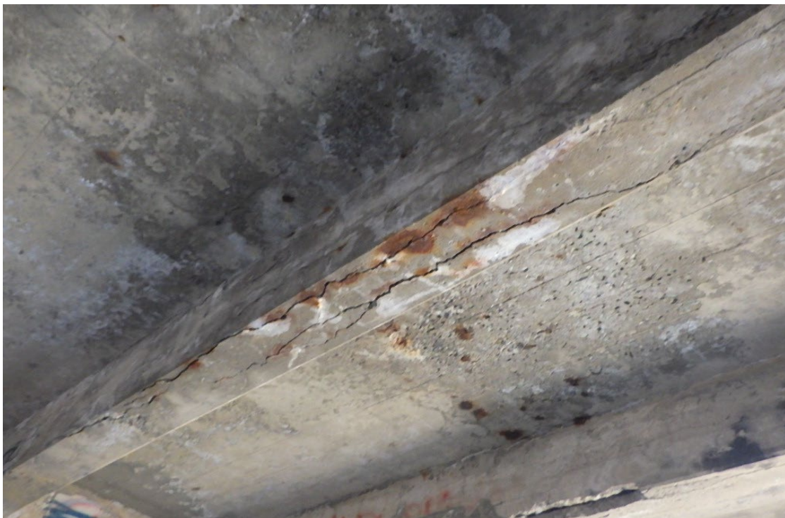
40. Cracks with rust and efflorescence and delaminated concrete in the bottom of Beam 3, Span 7.
