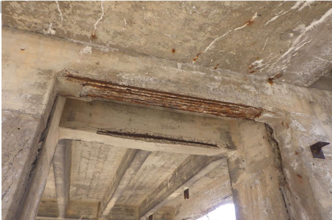
51. Spalls with exposed rebar in the cap at Pier 4.
