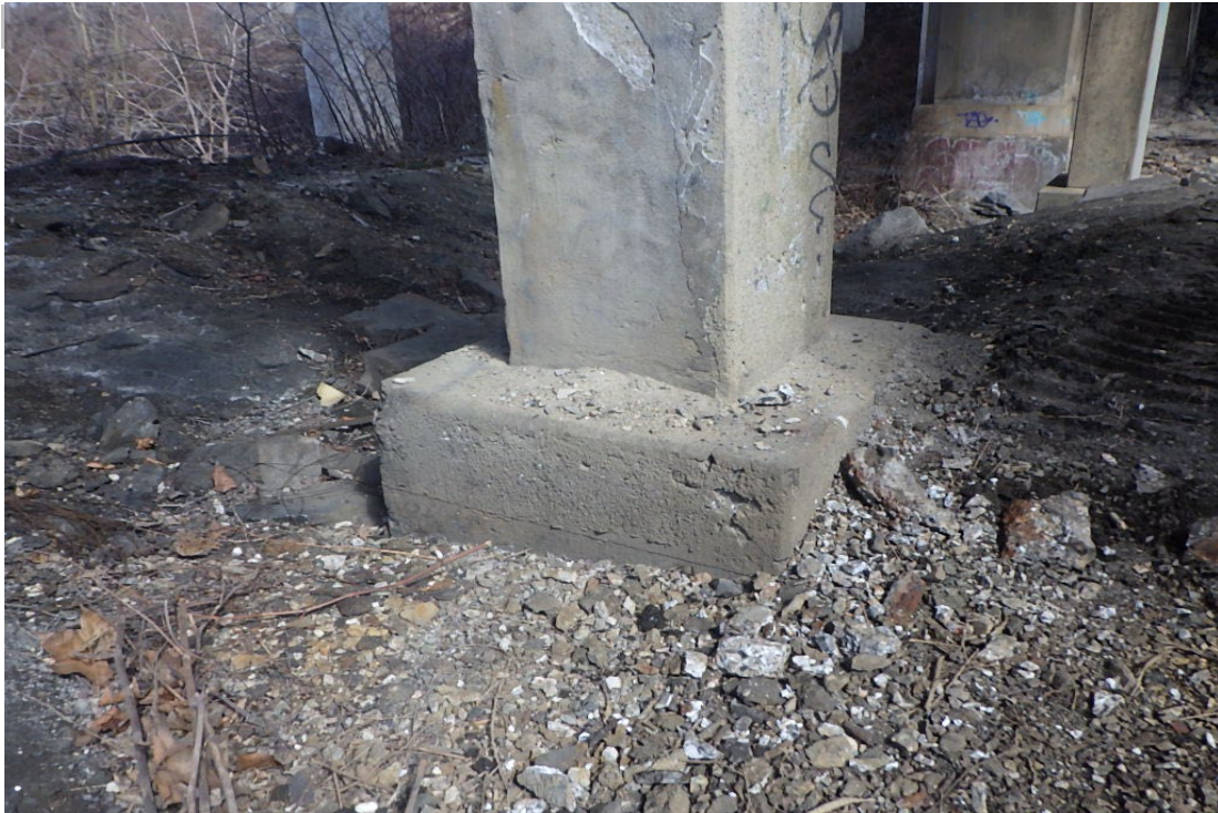
49. Exposed footings at Pier 3.
