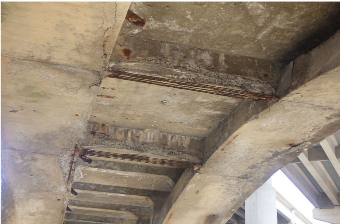
34. Floorbeams 5 and 6 in Span 5 with severe spalling across the bottom.
