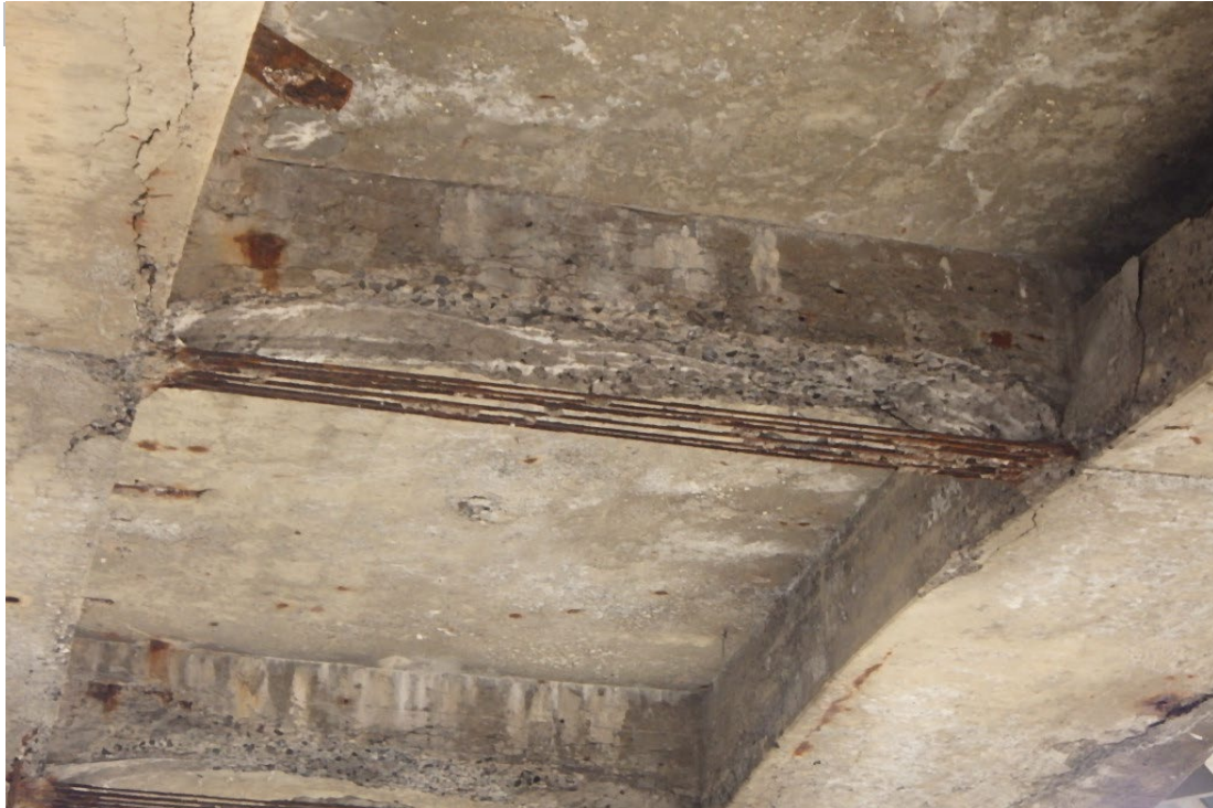
35. Close up of Floorbeam 5 with up to 12" gap between the concrete and bottom reinforcement.
