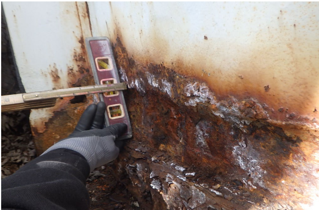
20. Advanced section loss to the bottom of the web of the right girder at the near end.
