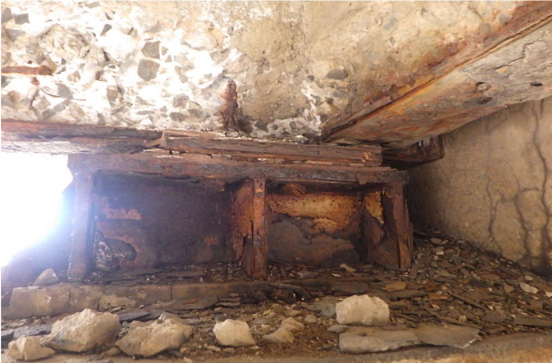
25. Girder bearings in Span 2 with heavy rust and pack rust. Note the bearings are frozen in expansion.
