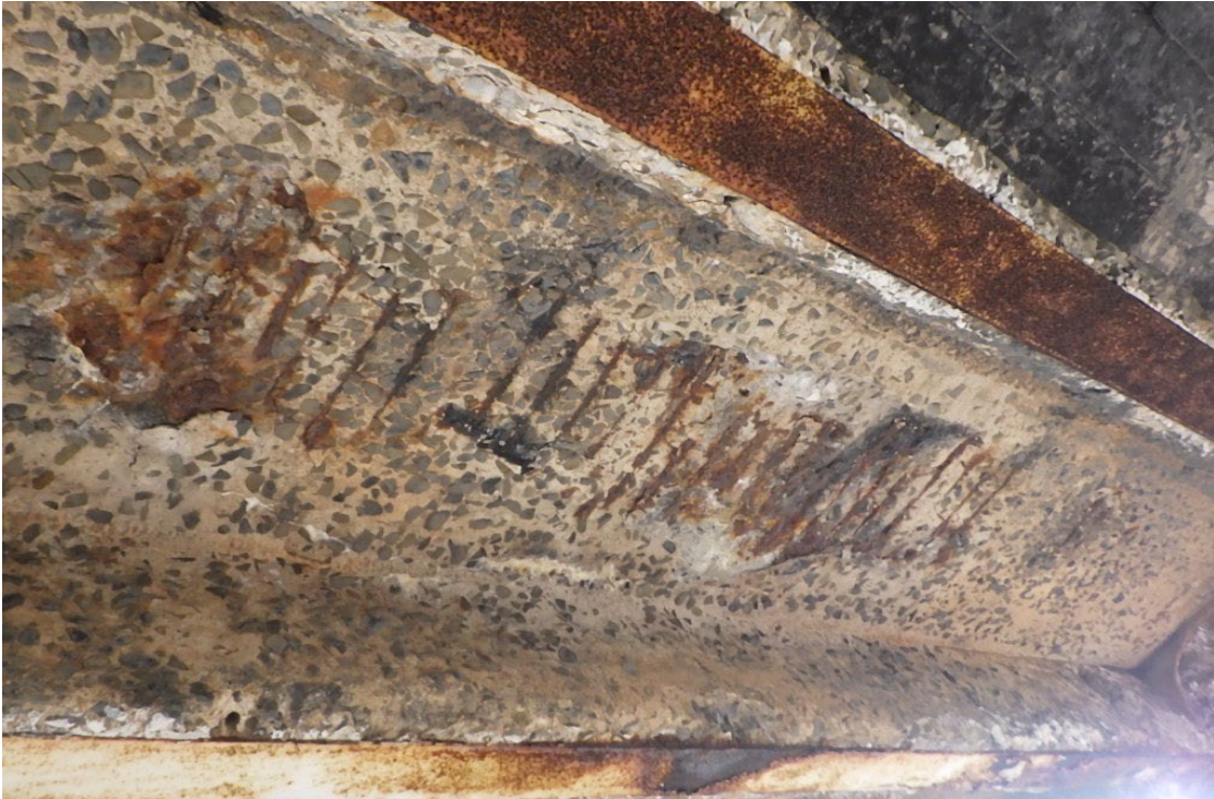
17. Spalls with exposed rebar in the underside of the deck in Span 2.
