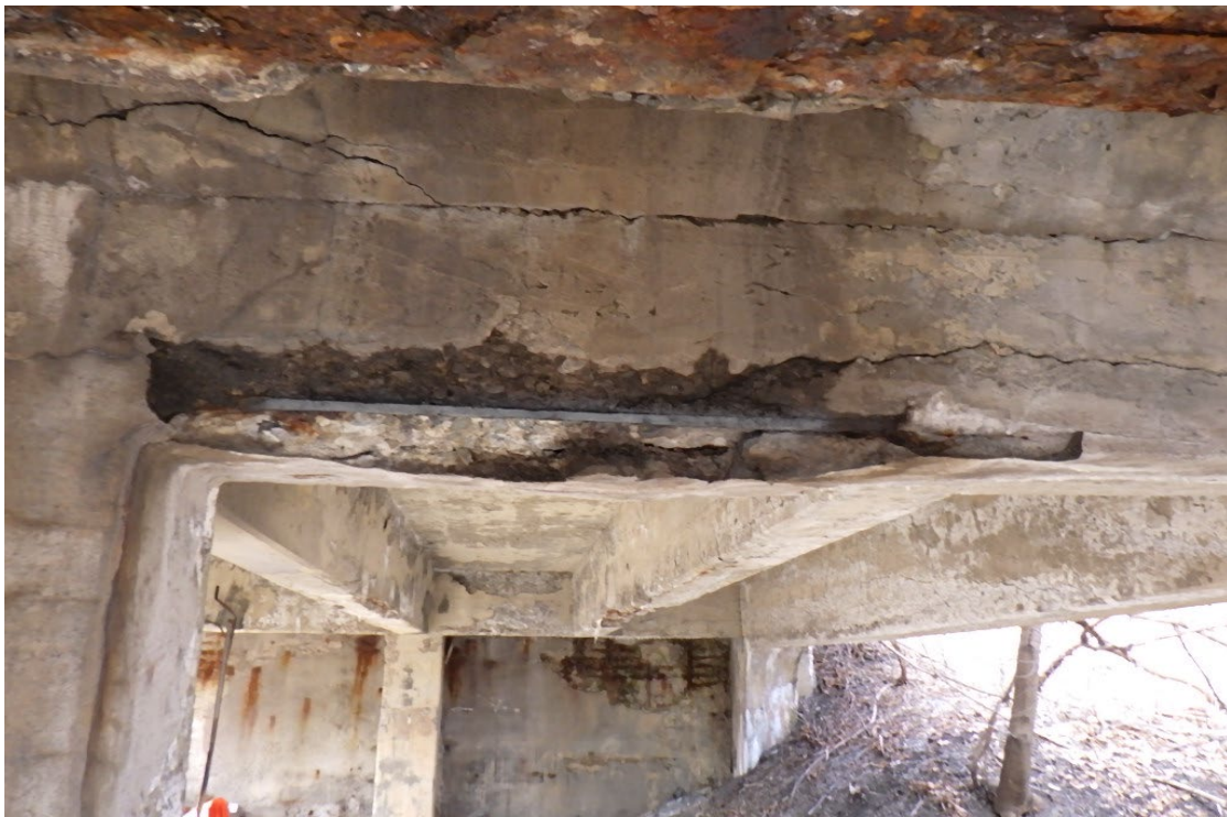
46. Spall with exposed rebar in the Pier 1 cap.
