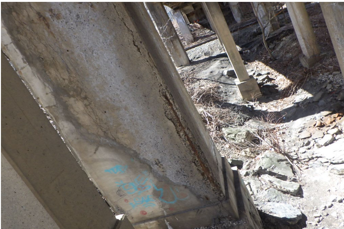
52. Spall with exposed rebar at the bottom of the right column at Pier 4.
