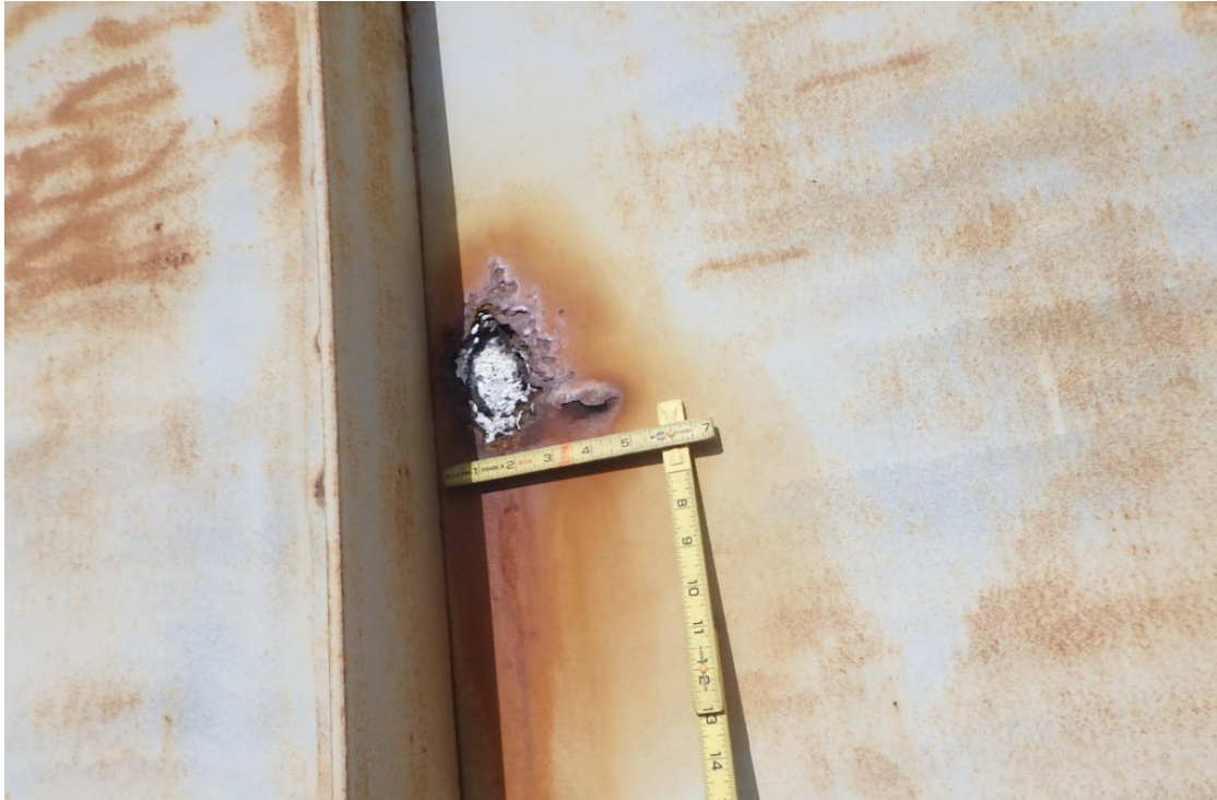
21. Newly noted hole in the Left Girder web at Floorbeam 13.
