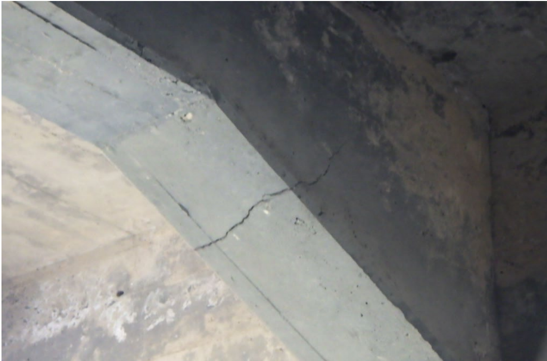
39. Shear crack in the haunches of the beams in Span 7.
