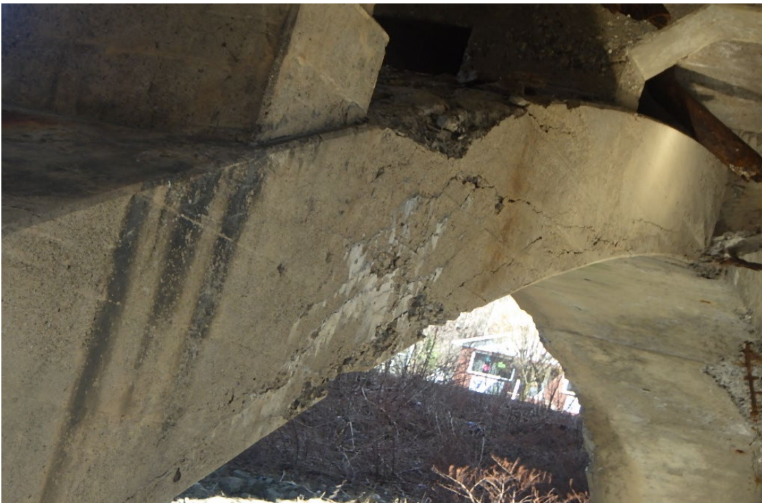
32. Cracks with delaminated concrete and spalling along the left arch rib.
