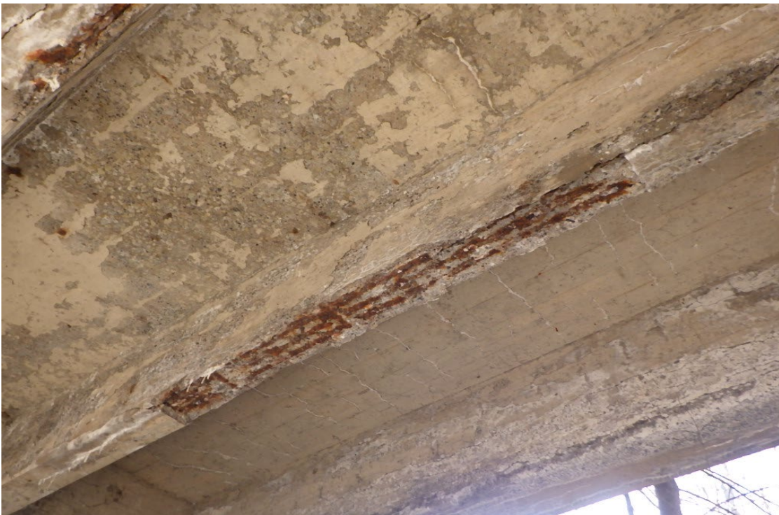
14. Beam 2, Span 1 with cracks, delamination and spalls with exposed rebar.
