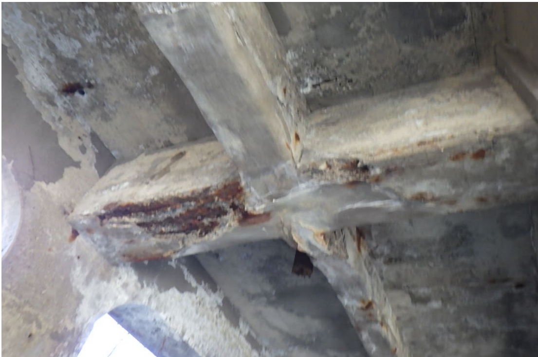
54. Spall with exposed rebar in the cap of Pier 6.
