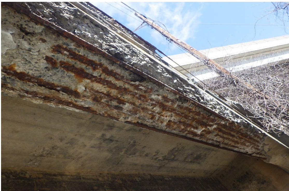
30. Beam 5 in Span 4 spall with six exposed longitudinal bars.
