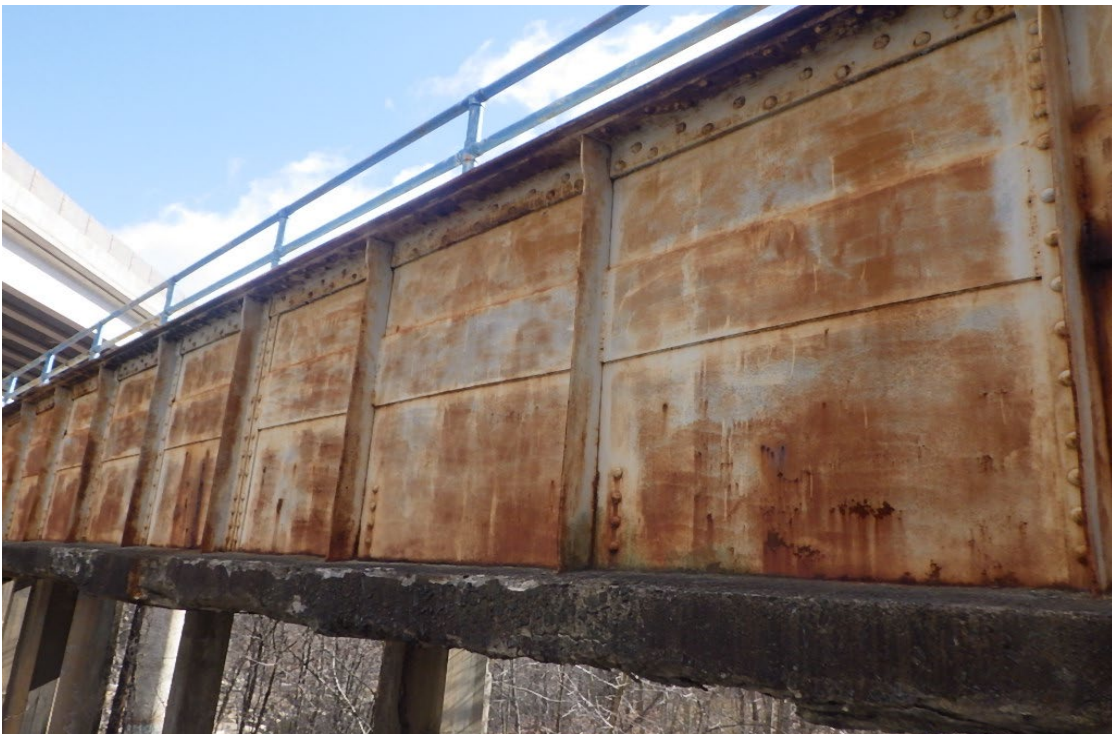
18. Typical moderate to heavy rust along the through girder webs.
