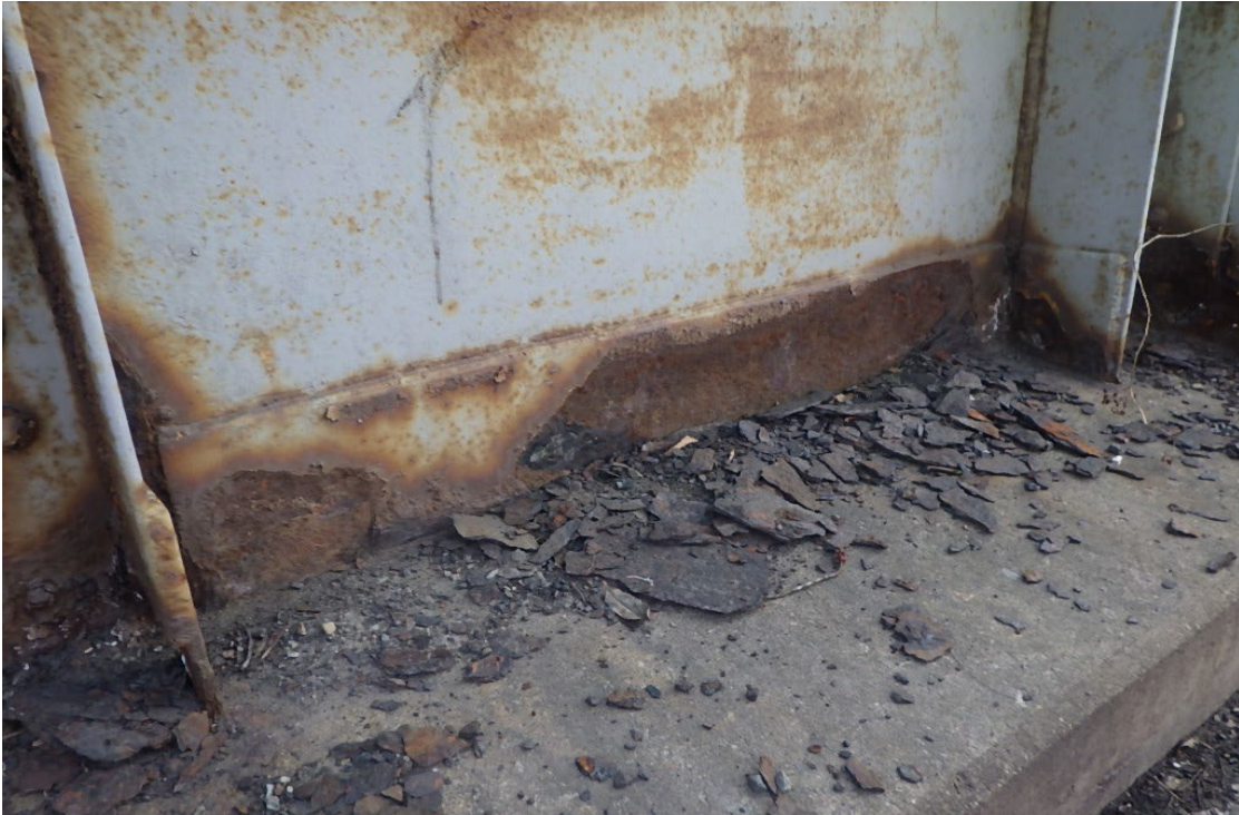
11. Typical section loss to the web plates along the Right Girder.
