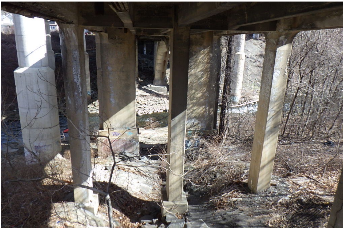
48. Typical pier for the T-beam spans. Pier 3 shown, looking ahead.
