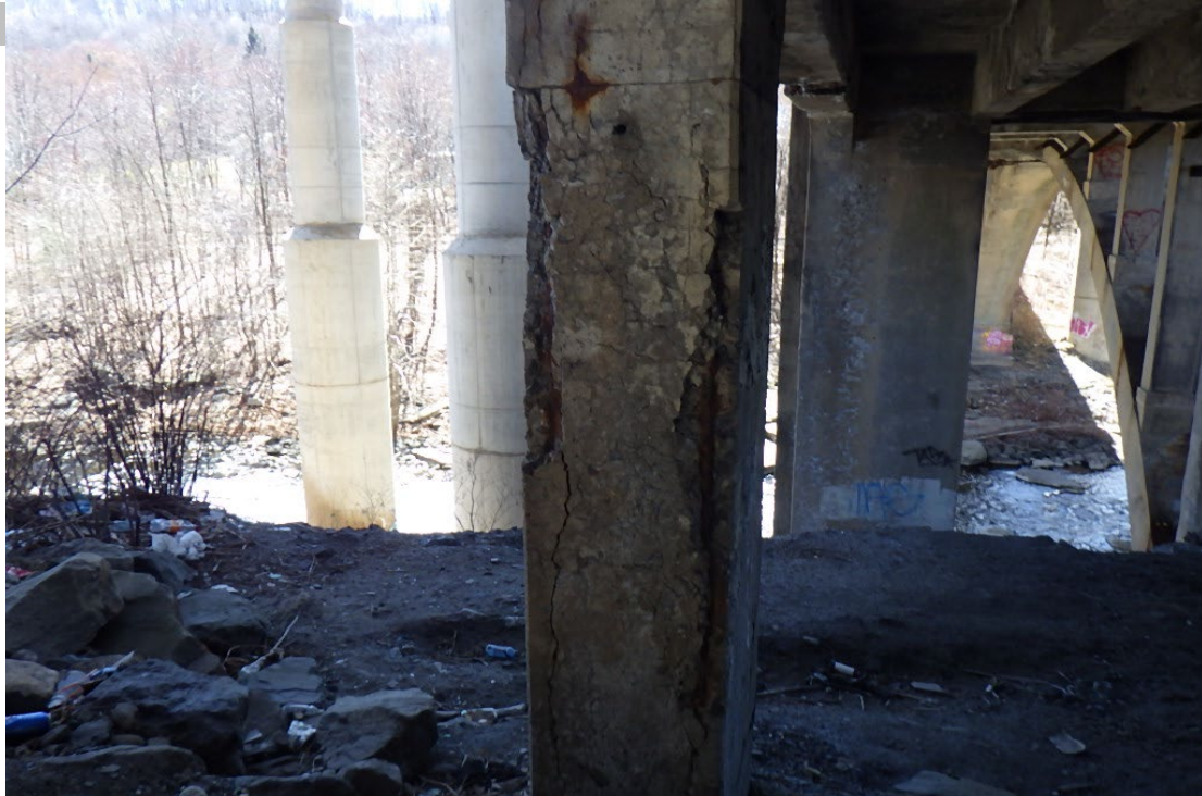
55. Cracks and spalls at the corners of Column 3 at Pier 6.
