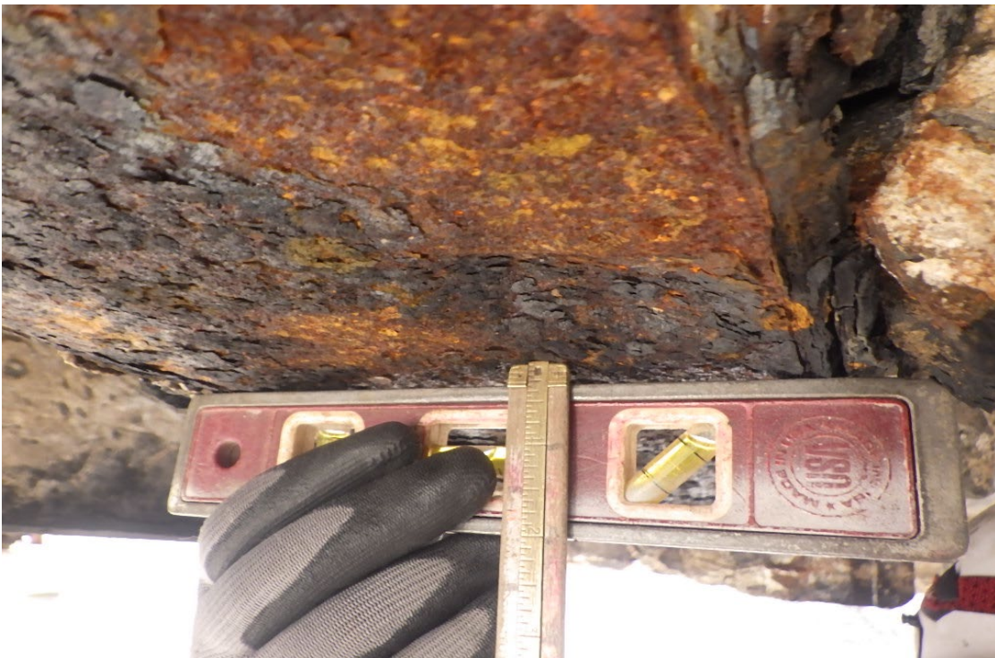
24. Section loss to the underside of the floorbeam bottom flanges.
