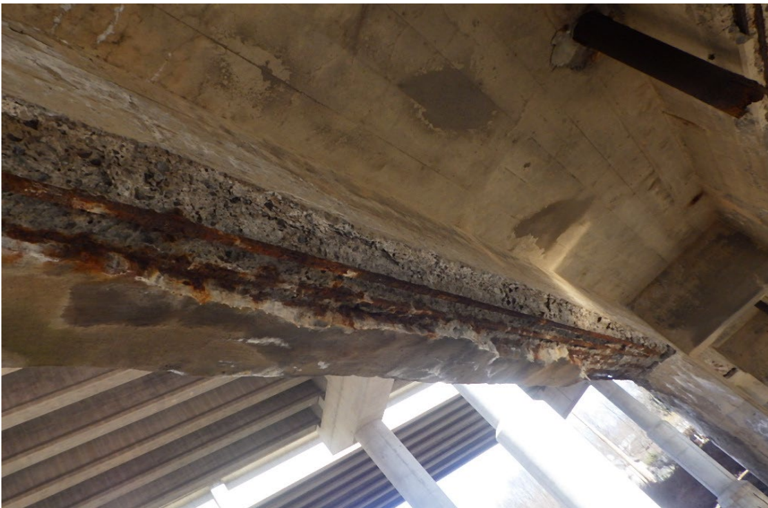
28. Span 3, Beam 1 spall throughout length with exposed and debonded rebar.
