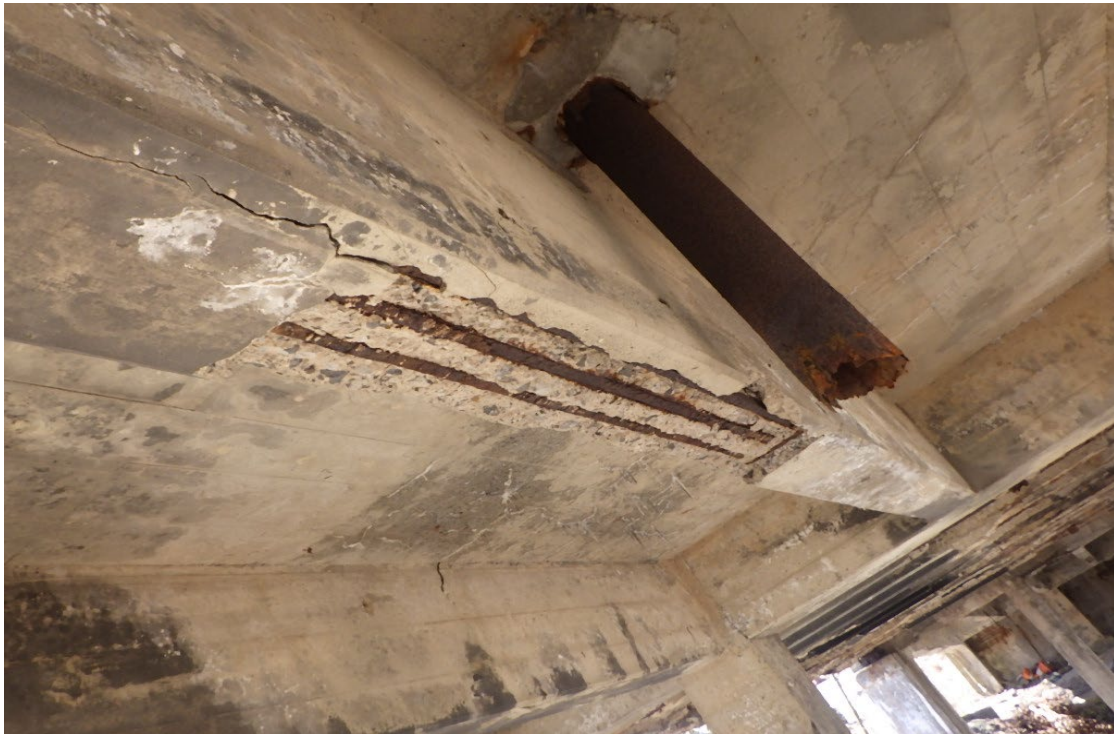
29. Spall with exposed rebar in the bottom of Beam 2 in Span 3.
